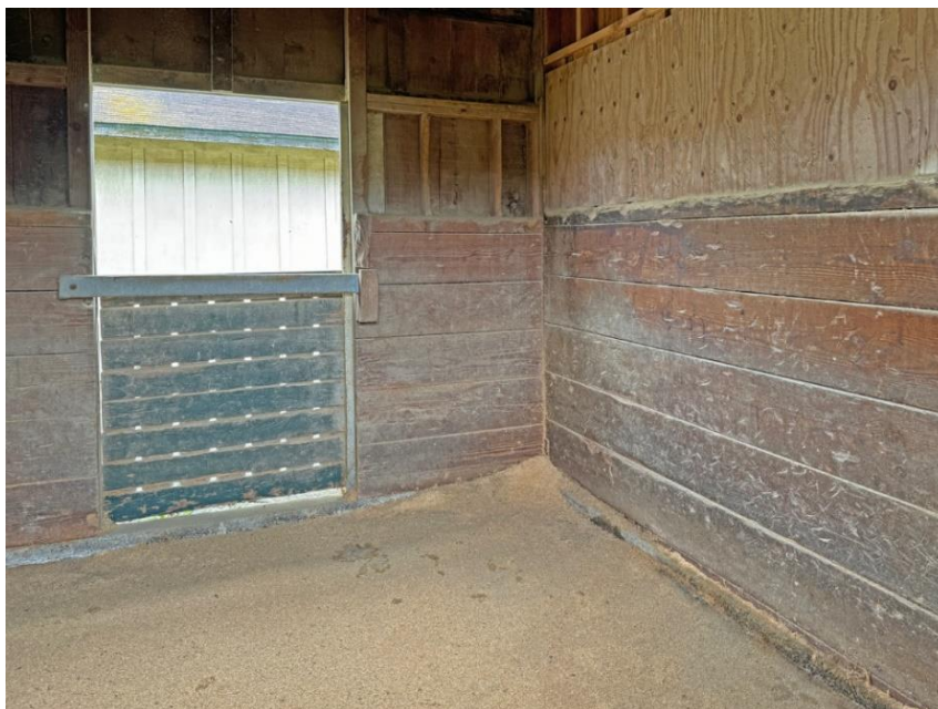
Photograph 15: View looking inside a typical stall with old growth redwood siding.
