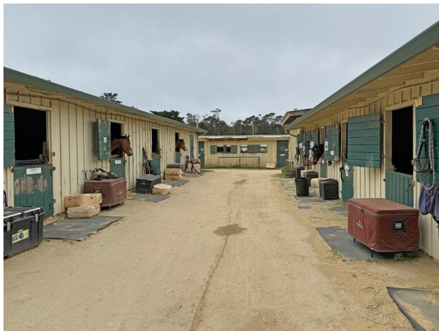
Photograph 13: View looking south at the aisle between the stables and stalls.
