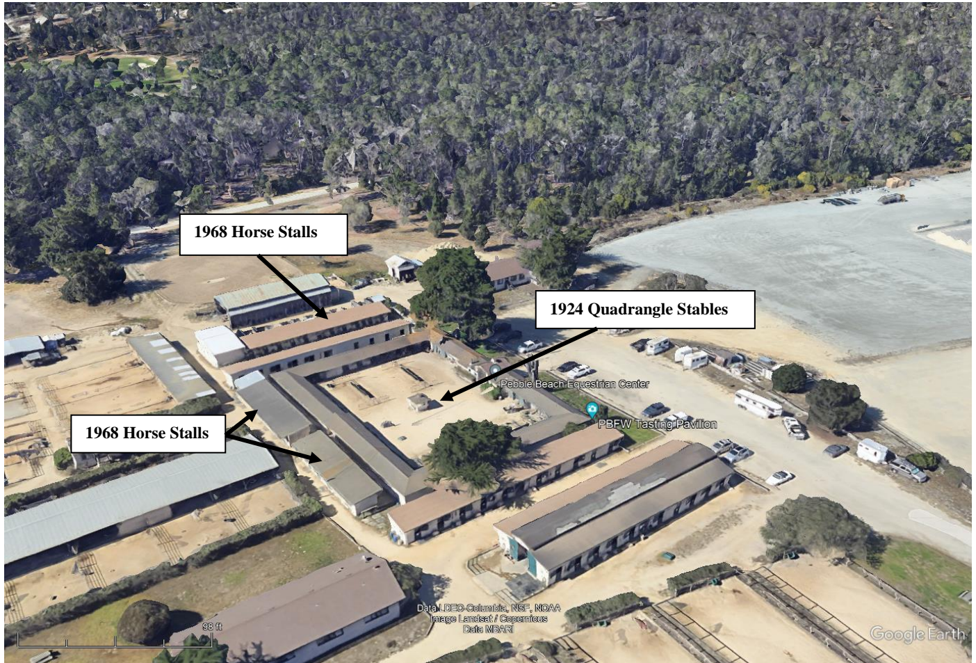
Figure 10: Aerial photograph of the significant buildings at PBEC.
