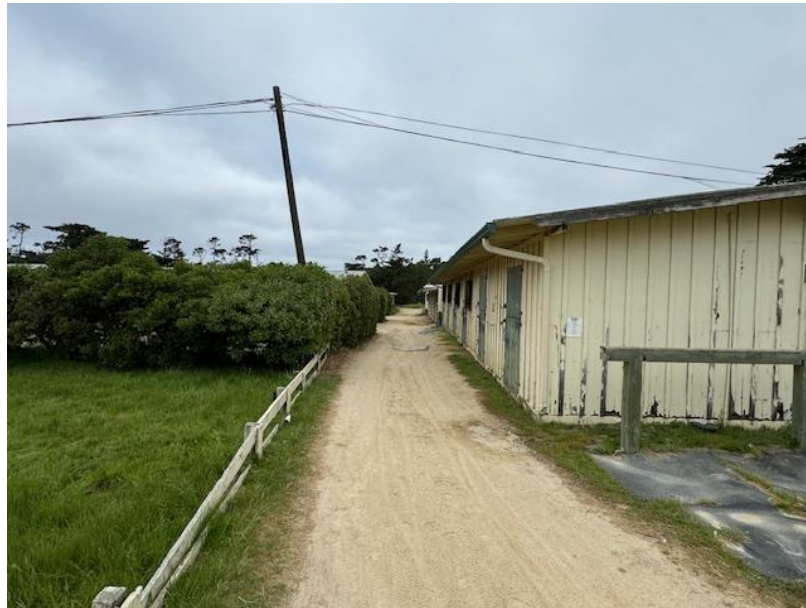
Photograph 16: View looking west at the 1968 horse stalls.
