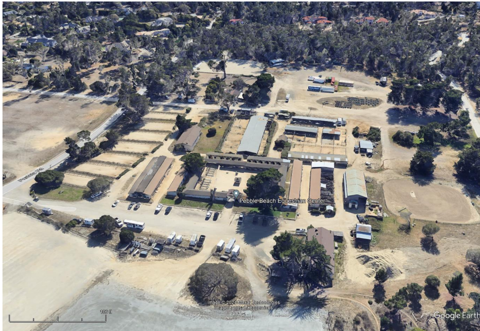
Figure 2: Aerial photograph of the PBEC looking southwest (Google Earth 2024).
