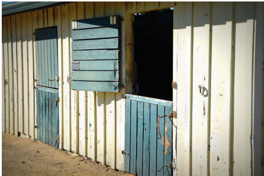
Photograph 12: Close-up of the 1924 stalls with Dutch doors and wood salvaged from the schooner Flavel.
