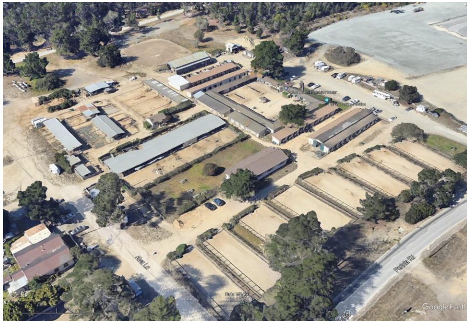
Figure 3: Aerial photograph of the PBEC looking north (Google Earth 2024).
