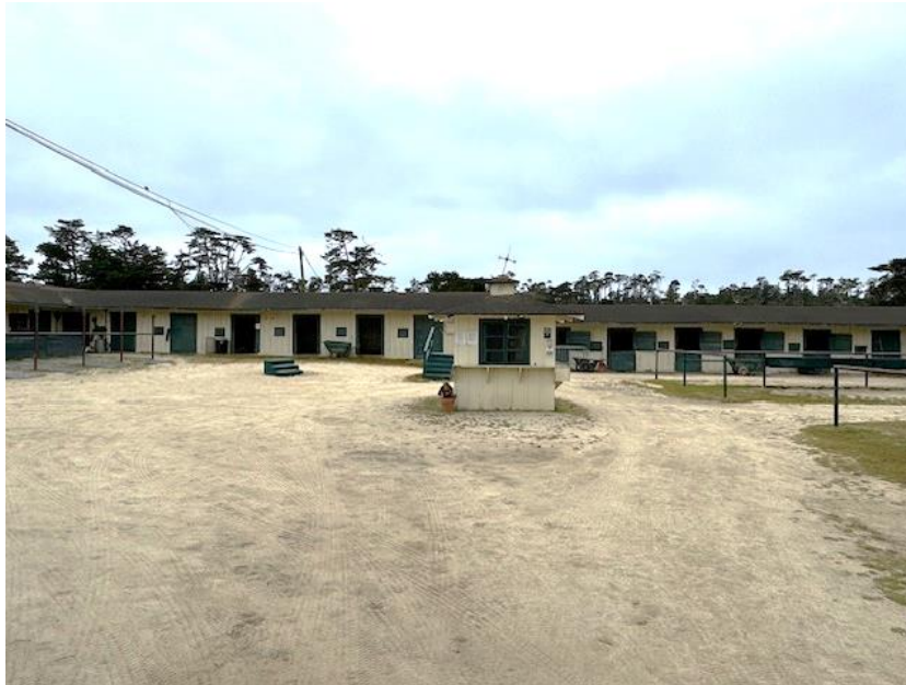
Photograph 10: View looking west inside the quadrangle stables and the kiosk.
