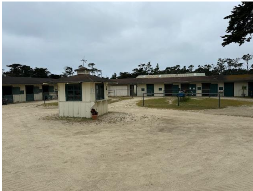
Photograph 11: View looking southwest inside the quadrangle stables and kiosk.
